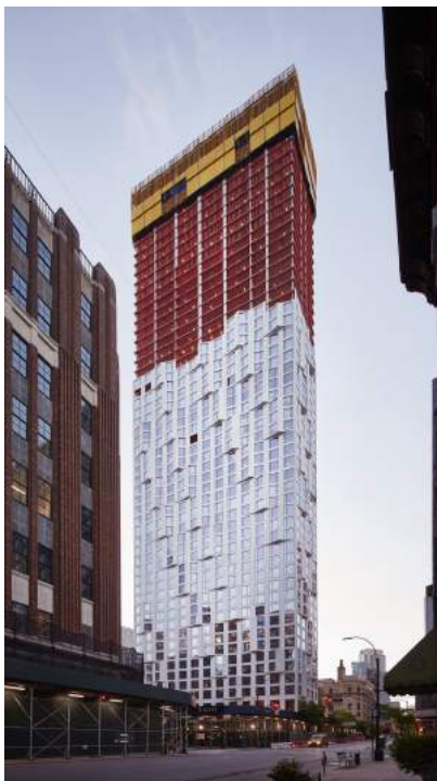
The topped-out construction of 11 Hoyt.
